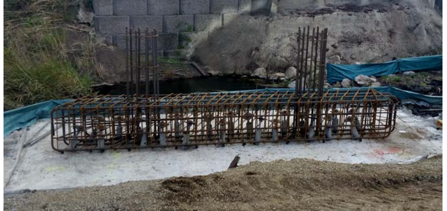
Micropiles installed in the central pier pile cap with column extensions for mid span headstock
