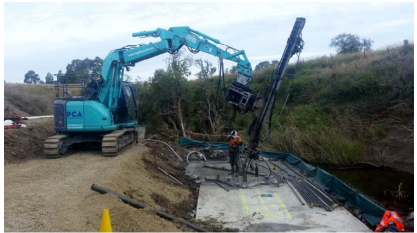
Installing micropiles in the central pier
