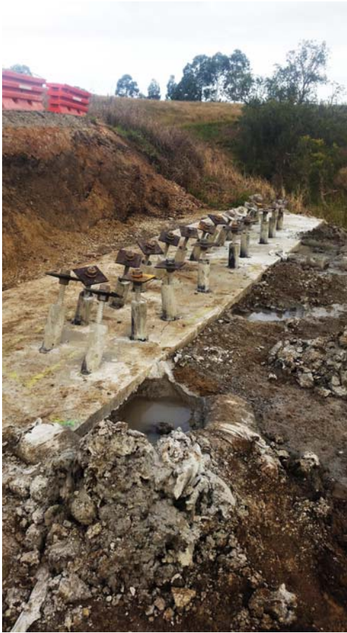
Micropiles installed in abutment prior to installation of reinforcing cage
